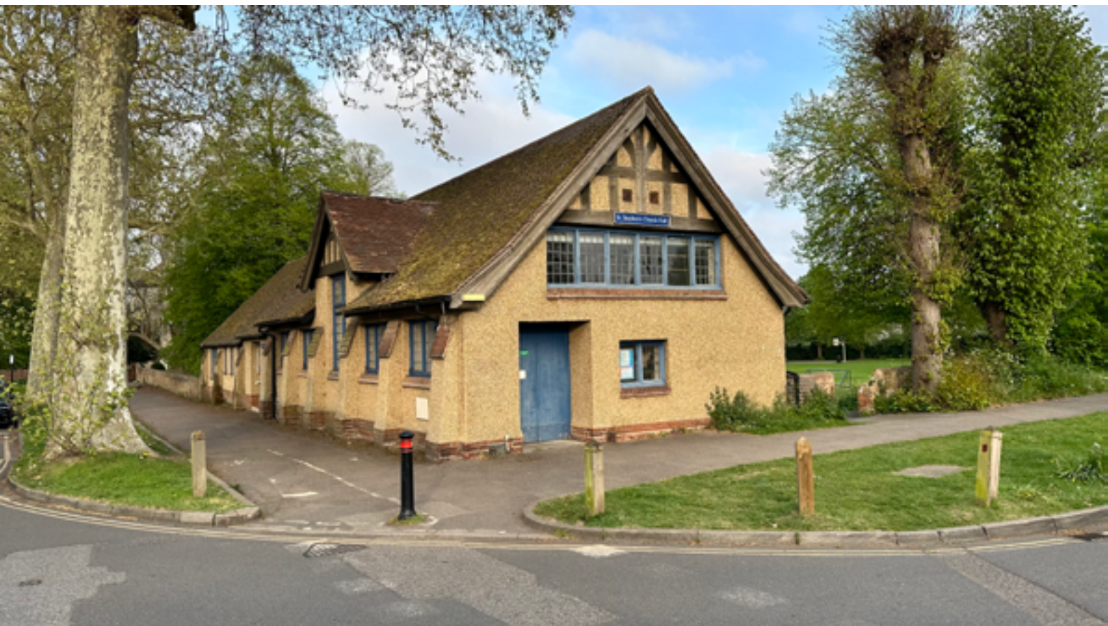
▲ St Stephen's Church Hall; the church is at the end of the path towards the left of this picture
